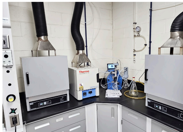
PC 3012 NT VARIO select vacuum pump installed within the lab.
